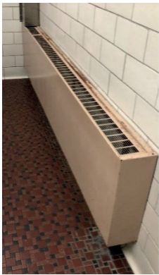
L - bathroom fintube. C - corridor fintube. R - entry vestibule convector.
