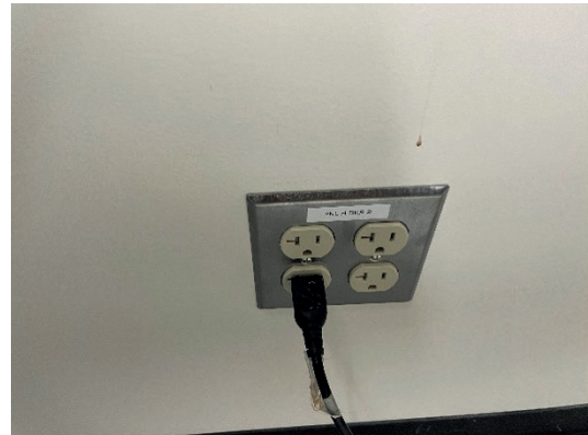
New Receptacle in New Wall
