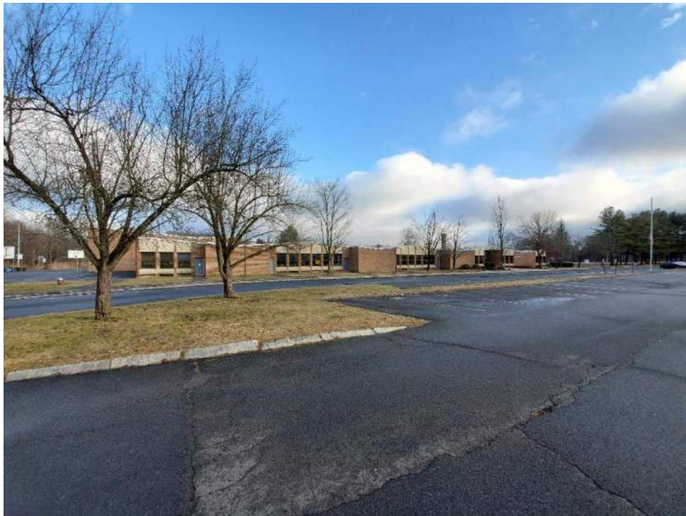
Photograph 2 – Fort River Elementary west side of building.
