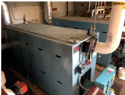
L- two cast iron oil fired boilers. C- Breechings with draft damper ties into existing masonry chimney. R- chimney and chiney cap on roof.
