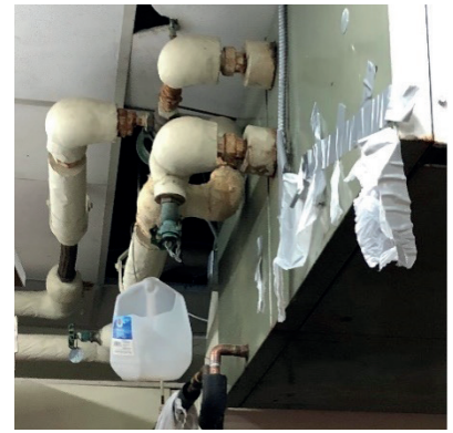
L & C - Other original vintage indoor AHUs, horizontal type. R - this particular one has some duct tape to keep together, and note the ACM insulation on pipe elbows.
