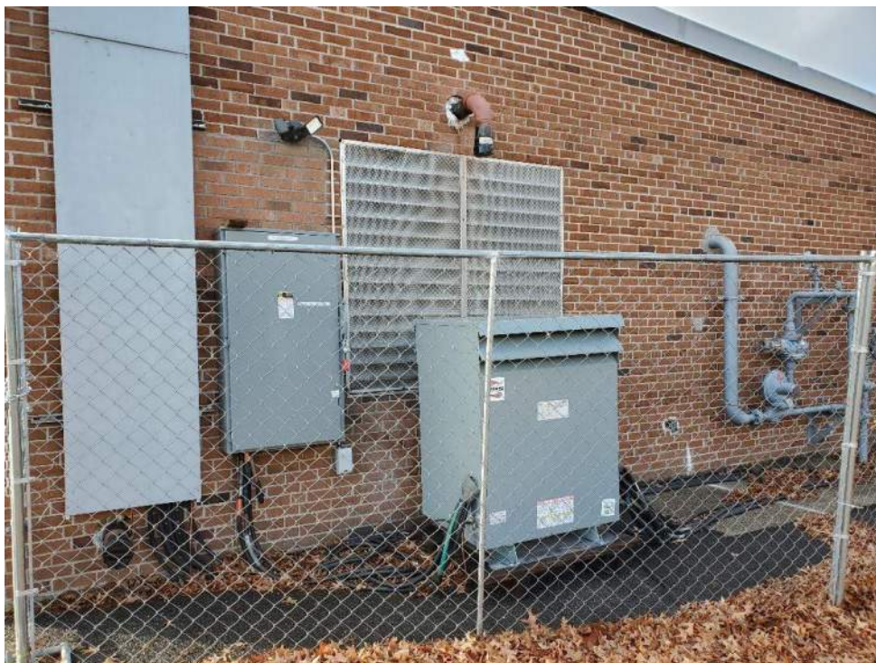
Photograph 6 – Mechanical hookups on south side of building.
