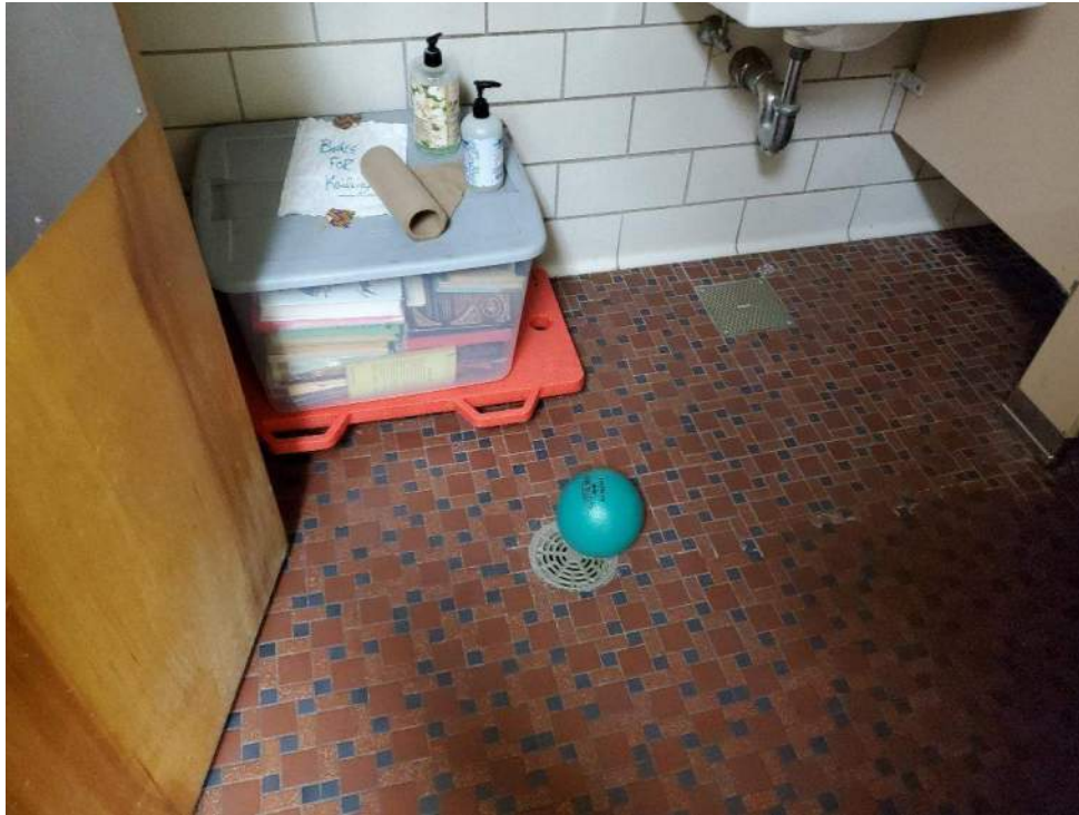
Photograph 19 – Typical bathroom floor drain.
