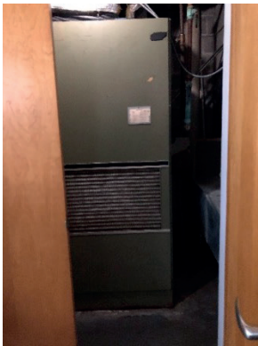
Typical original vintage vertical indoor Trane air handling unit.
