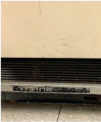
L & C - Classrooms have original vintage Trane unit ventilators. R - unit ventilator fresh air intake louvers are just few inches from the ground level, here shown at pavements but most are above grass areas where they are prone to grass clipping ingestions, resulting in plugged intake screens.
