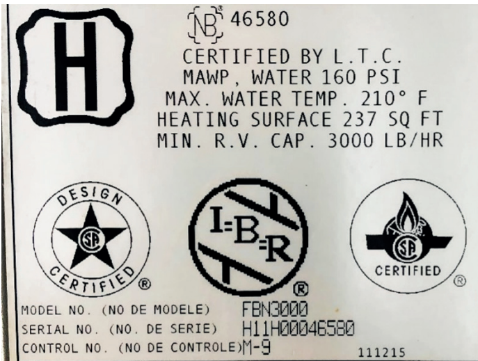
Lochinvar Crest Boiler nameplates serial number H11H00046590 show that they were manufactured in August 2011 (11 years ago), and model number FBN3000 indicates 3.0 million BTUH input.
