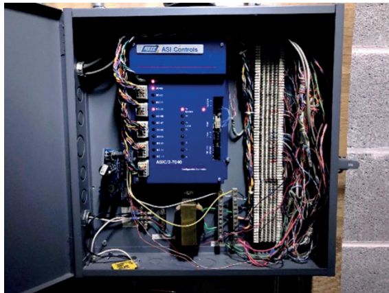
L - DDC controllers, showing that some parts of the controls have been modified. R - original vintage pneumatic thermostats are throughout the school.
