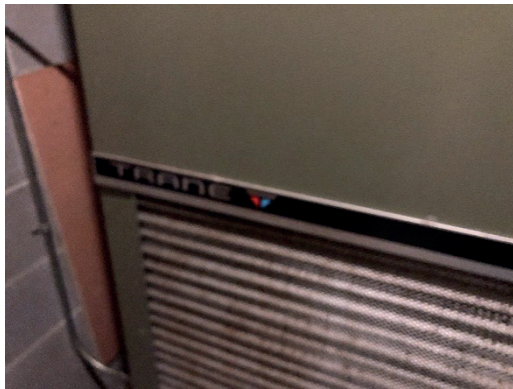
Typical original vintage vertical indoor Trane air handling unit.
