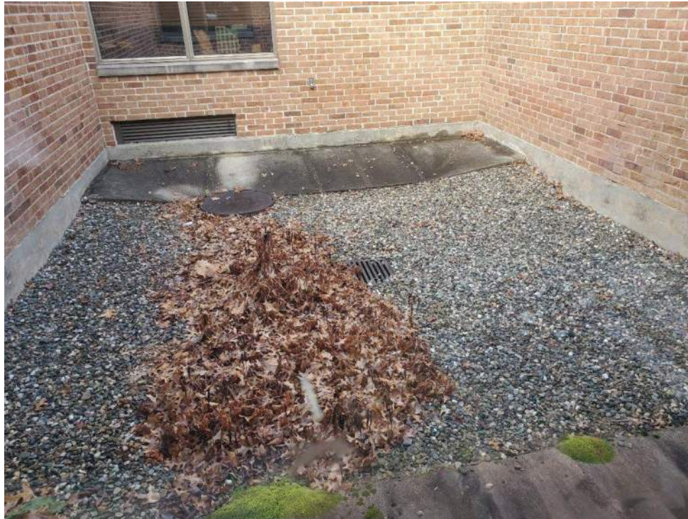
Photograph 15 – Quad courtyard catch basin.
