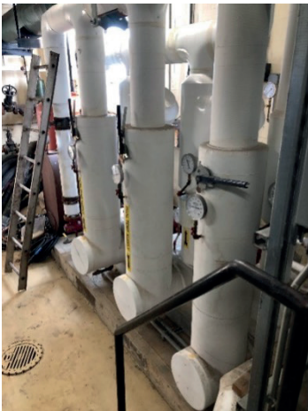
Four dual-temperature circulating pumps, appears to have been installed at the same time as the boilers.
