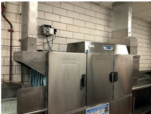
L - dishwasher. R - note the feeder table disposal and backflow preventor.
