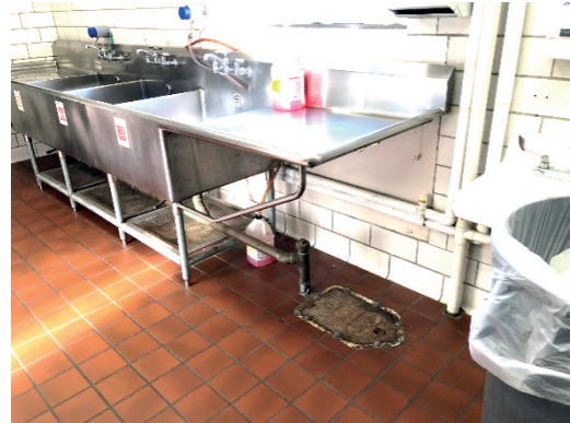
L - Pot sink #1 with disposal. R - Pot sink #2 with grease trap under slab which can be serviced.
