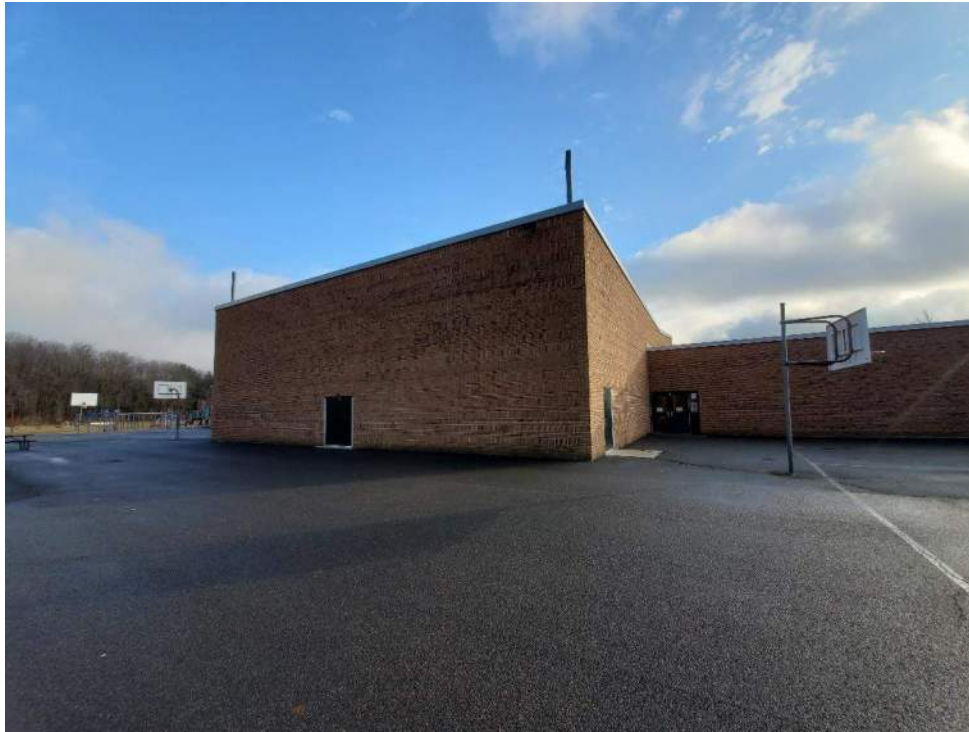
Photograph 3 – Fort River Elementary north side of building.
