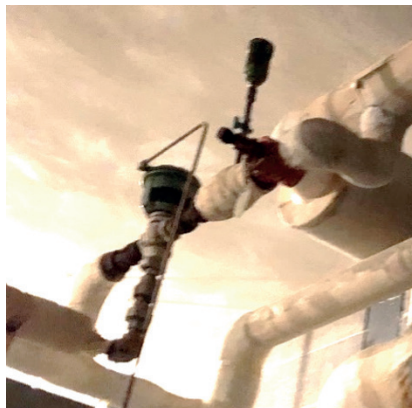
L & C - pneumatic control valves. R - pneumatic control damper.
