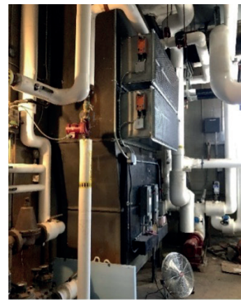
L- A set of 4" lines are extended to outside for temporary chiller hookup in case of chiller failure. R- boiler combustion air duct; lower opening had to be blocked off to prevent freezing.
