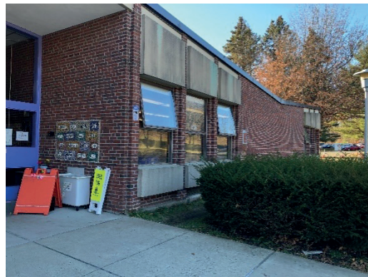
L- unit ventilator intake louver is just a few inches above ground, prone to grass and debris ingestion; leading to plugged up screens. R- many windows were opened during the cold day.
