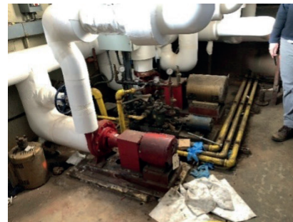
Pumps - main dual temperature duplex B&G 310 GPM @95' head. High temperature loop 140 GPM at 95' head. High temperature water for cafeteria and DHW 20 GPM @ 30' head.
