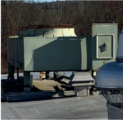
L - original 49 year old air cooled condensing unit on roof failed last year. C - note temporary electrical power cables on roof which were ran from the chiller to the rental chiller; nameplate was illegible, but thought to be 70-tons, which would be considered severely undersized by today's standard. R - chiller barrel (black above white pipes) inside right below.
