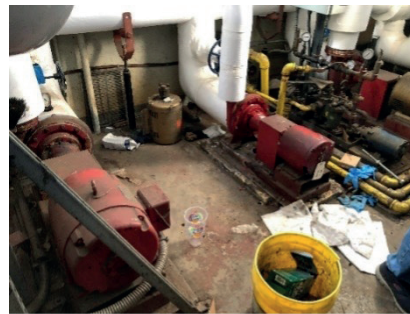
L - a 10,000-gallon underground fuel oil storage tank just outside the boiler room serves the space heating boilers; a 280-gallon underground tank serves the generator. C - Veeder-Root fuel oil level meter. R - fuel oil transfer pump set.
