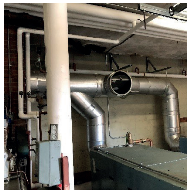
L- two cast iron oil fired boilers. C- Breechings with draft damper ties into existing masonry chimney. R- chimney and chiney cap on roof.
