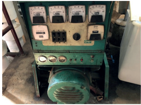
Small Onan diesel generator- mechanical component is its fuel system. air louvers, and exhaust stack.
