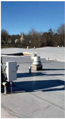
Original vintage roof exhaust fans.
