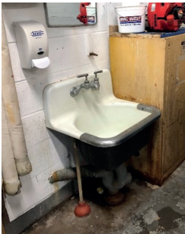
Janitors sink and Can Washer.
