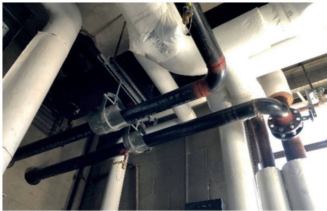
L- A set of 4" lines are extended to outside for temporary chiller hookup in case of chiller failure. R- boiler combustion air duct; lower opening had to be blocked off to prevent freezing.
