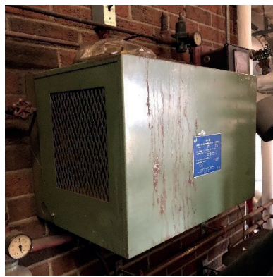
L - pneumatic control air compressor. C - pneumatic air dryer. R - Original pneumatic control panel.
