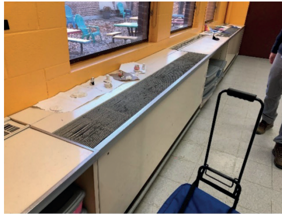
L & C - Classrooms have original vintage Trane unit ventilators. R - unit ventilator fresh air intake louvers are just few inches from the ground level, here shown at pavements but most are above grass areas where they are prone to grass clipping ingestions, resulting in plugged intake screens.
