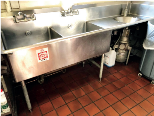
L - Pot sink #1 with disposal. R - Pot sink #2 with grease trap under slab which can be serviced.
