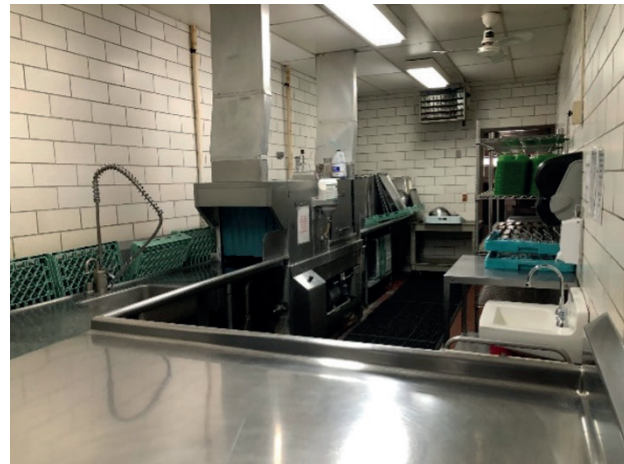
L - only means of heat in the kitchen is this hot water unit heater. R - dishwasher, and exhaust ducts up.
