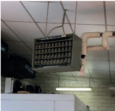
L - only means of heat in the kitchen is this hot water unit heater. R - dishwasher, and exhaust ducts up.
