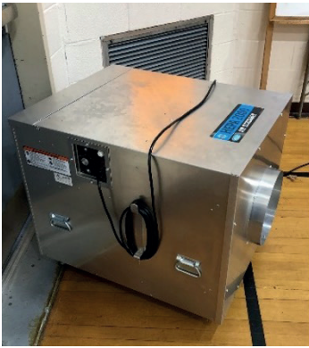
L - large portable HEPA filter unit in Gym. R - smaller and quieter portable HEPA filter units were found throughout the school.
