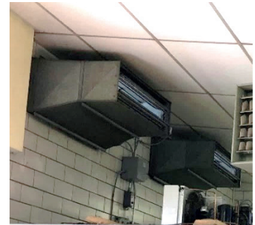
L & C- kitchen cooking line exhaust hood; the filters are Code- compliant panel type, but does not have Code mandated Ansul system. R- make up air is untreated (filtered or heated) through intake louver... understandably during summer it is hot and humid, but during winter the kitchen becomes freezing cold.
