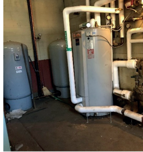
L - Water service comprising of water meter and pressure regulator, suggesting that they have more than 80 psig feed. Note that there is not backflow preventor. R - indirect domestic hot water heater.
