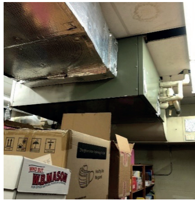
L & C - Other original vintage indoor AHUs, horizontal type. R - this particular one has some duct tape to keep together, and note the ACM insulation on pipe elbows.
