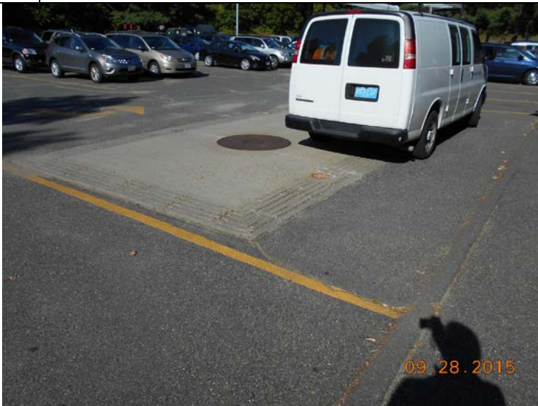
Photo #7: UST pad shown
