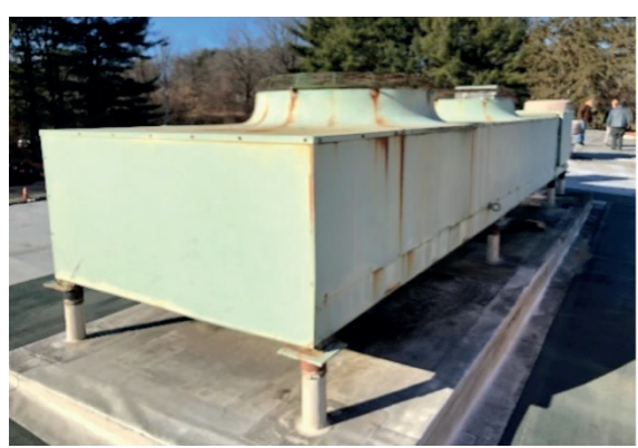
L- original 52 year old air cooled condensing unit on roof, still works most times; nameplate was illegible, but thought to be 70-tons, which would be considered severely undersized by today's standard. R- chiller barrel (black above white pipes) inside right below.
