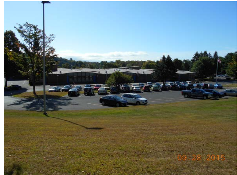
Photo #2: View from north
