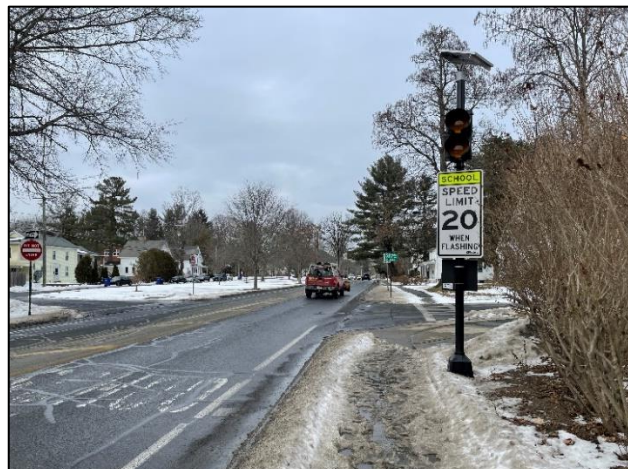
Photo 5: Flashing school speed signs on South East Street are not functioning.
