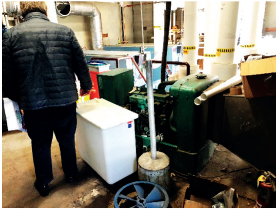
Small Onan diesel generator- mechanical component is its fuel system. air louvers, and exhaust stack.
