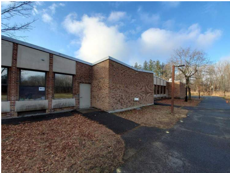
Photograph 4 – Fort River Elementary northeast side of building.
