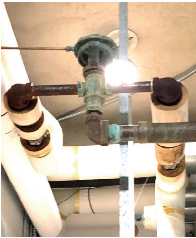
L - pneumatic control valve, here with ACM insulation sections removed. C - pneumatic control valve, here with remnants of encapsulated ACM insulation remaining. R - Electronic damper actuator.
