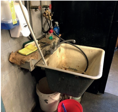
Janitors sink, Mop Receptor, and Can Washer.
