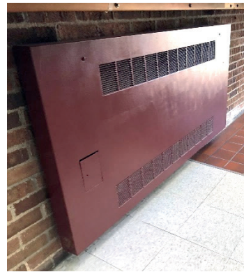
L & C - Classrooms have original vintage Trane unit ventilators. R - unit ventilator fresh air intake louvers are just few inches from the ground level, here shown at pavements but most are above grass areas where they are prone to grass clipping ingestions, resulting in plugged intake screens.
