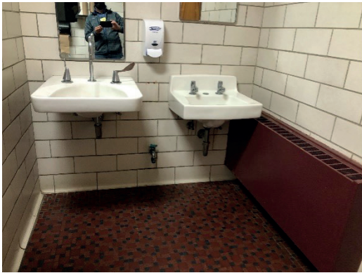
L - Pot sink #1 with disposal. R - Pot sink #2 with grease trap under slab which can be serviced.
