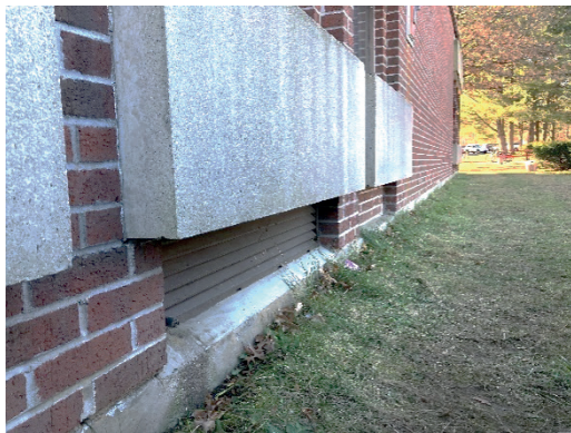
L- unit ventilator intake louver is just a few inches above ground, prone to grass and debris ingestion; leading to plugged up screens. R- many windows were opened during the cold day.
