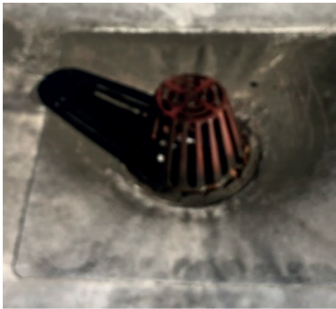
L- roof drain does not have overflow, are connected to internal conductor pipe, and to the under-slab piping to outside the building. R- roof edge does not have parapet.
