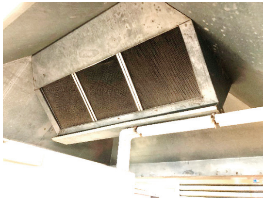
L - kitchen cooking line exhaust hood; the filters are non-Code-compliant mesh type, and does not have Code mandated Ansul system. R - make up air is untreated (filtered or heated) through intake louver... understandably during summer it is hot and humid, but during winter the kitchen becomes freezing cold.
