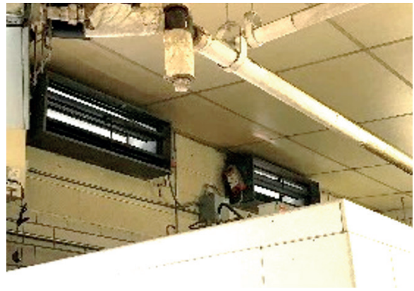
L - kitchen cooking line exhaust hood; the filters are non-Code-compliant mesh type, and does not have Code mandated Ansul system. R - make up air is untreated (filtered or heated) through intake louver... understandably during summer it is hot and humid, but during winter the kitchen becomes freezing cold.
