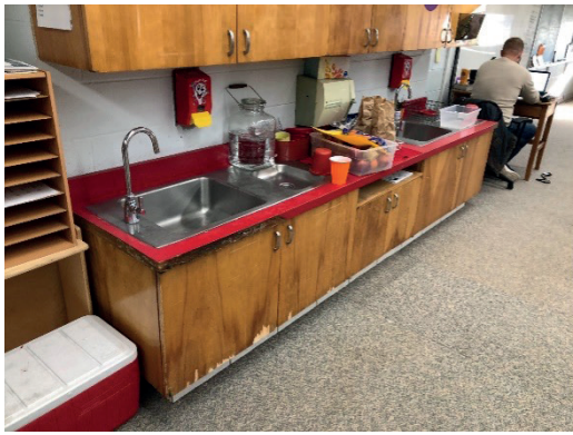
Inspection of several sinks showed that pipes were recently replaced.
