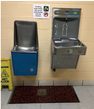
Accessible water coolers and bottle fillers.
