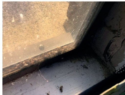
L- one of several courtyard/ lightwell. R- original single pane glass were retrofitted with plastic panel inside, apparently not tight so the insets are visible in the air space.
