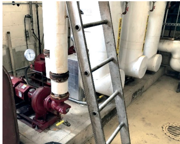
Four dual-temperature circulating pumps, appears to have been installed at the same time as the boilers.
