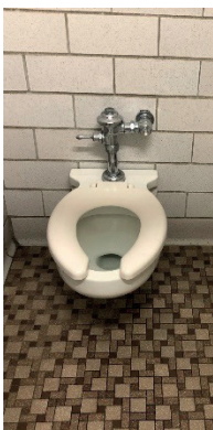
Fixtures are in fair shape, but not all bathrooms have accessible fixtures.
