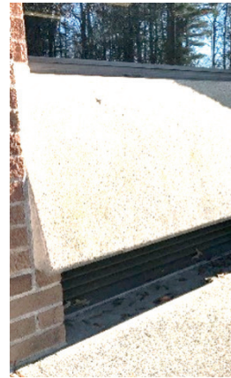
L & C - Classrooms have original vintage Trane unit ventilators. R - unit ventilator fresh air intake louvers are just few inches from the ground level, here shown at pavements but most are above grass areas where they are prone to grass clipping ingestions, resulting in plugged intake screens.
