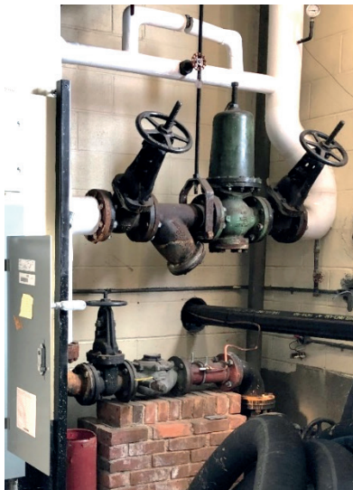
L - Water service comprising of water meter and pressure regulator, suggesting that they have more than 80 psig feed. Note that there is no Code mandated backflow preventor. R - indirect domestic hot water heaters.
