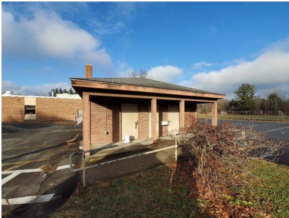
Photograph 8 – Recreational bathroom south of building.
