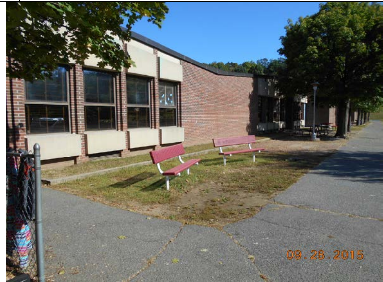
Photo #4: South side of school
