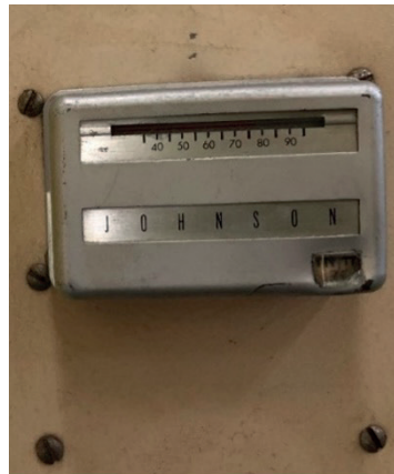
L - DDC controllers, showing that some parts of the controls have been modified. R - original vintage pneumatic thermostats are throughout the school.
