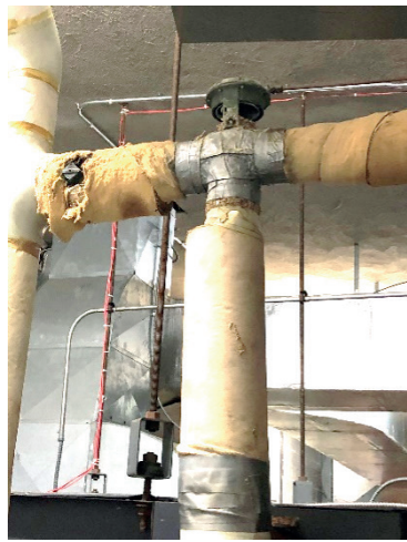
L - pneumatic control valve, here with ACM insulation sections removed. C - pneumatic control valve, here with remnants of encapsulated ACM insulation remaining. R - Electronic damper actuator.
