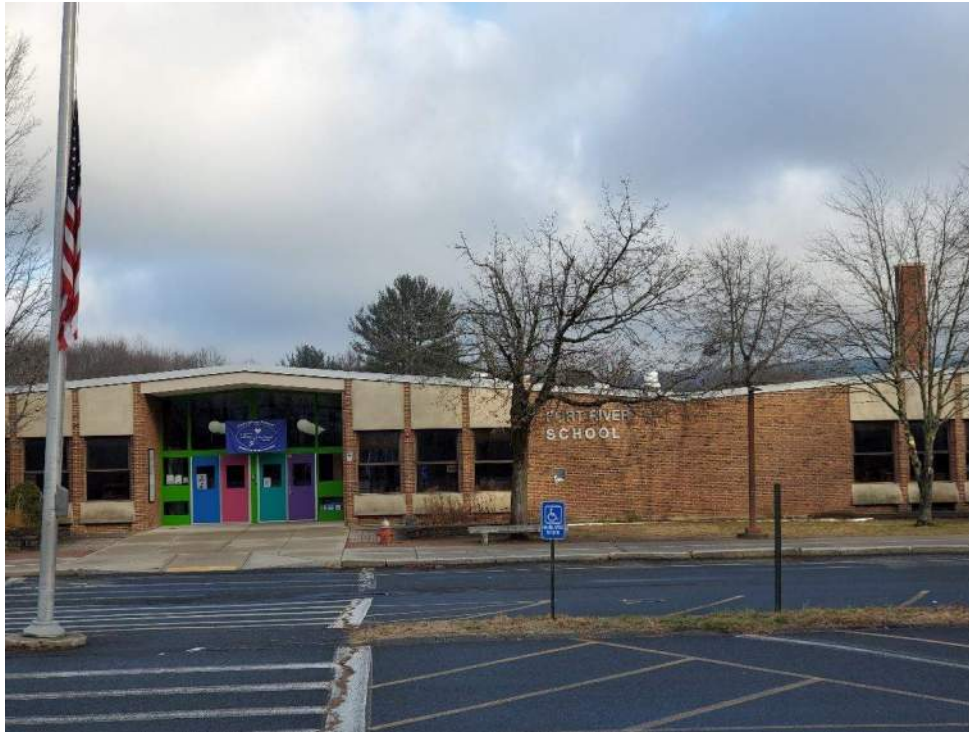
Photograph 1 – 70 S. East Street - Fort River Elementary School.
