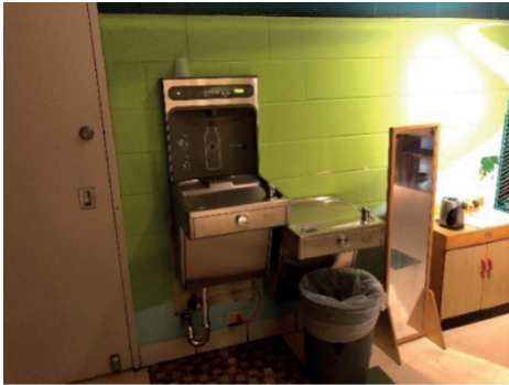
Accessible water coolers and bottle fillers.
