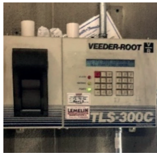
L - a 10,000-gallon underground fuel oil storage tank just outside the boiler room serves the space heating boilers; a 280-gallon underground tank serves the generator. C - Veeder-Root fuel oil level meter. R - fuel oil transfer pump set.
