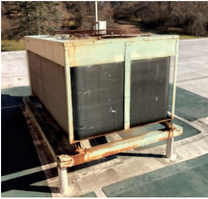
Original vintage air cooled condensing units, which amazingly are still operational, though doubtful reliably or with anyway near the full capacity.
