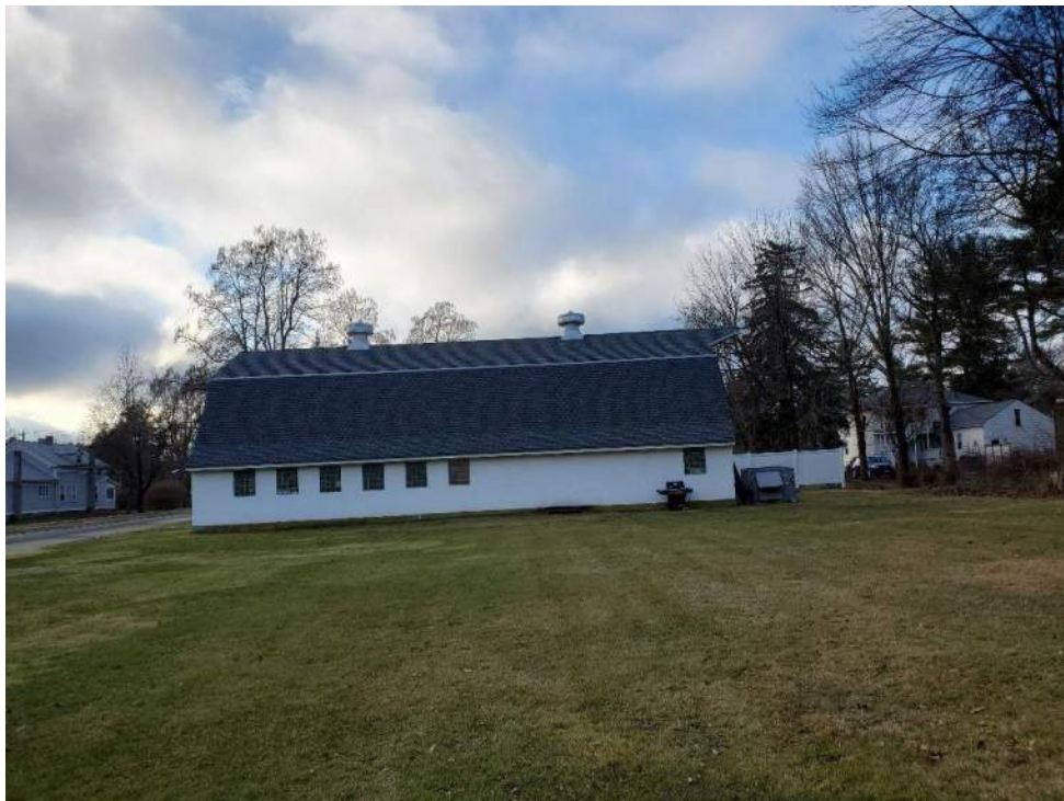
Photograph 34 – Storage facility on southwest portion of property (no access given).
