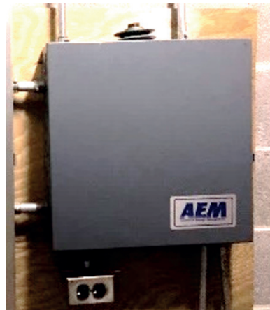
L - at least one of the control panel shows E-P (electronic- pneumatic) transducers, suggesting that DDC conversion, at least part, was made using the original pneumatic actuators. R - AEM DDC control panels.
