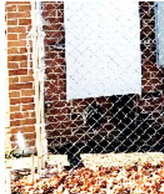
L & C - A set of 4" lines are extended to outside for temporary chiller hookup in case of chiller failure. R- boiler combustion air duct, which is no longer needed since the new boilers bring in outside air through individual ducts.
