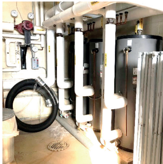
L - Water service comprising of water meter and pressure regulator, suggesting that they have more than 80 psig feed. Note that there is no Code mandated backflow preventor. R - indirect domestic hot water heaters.
