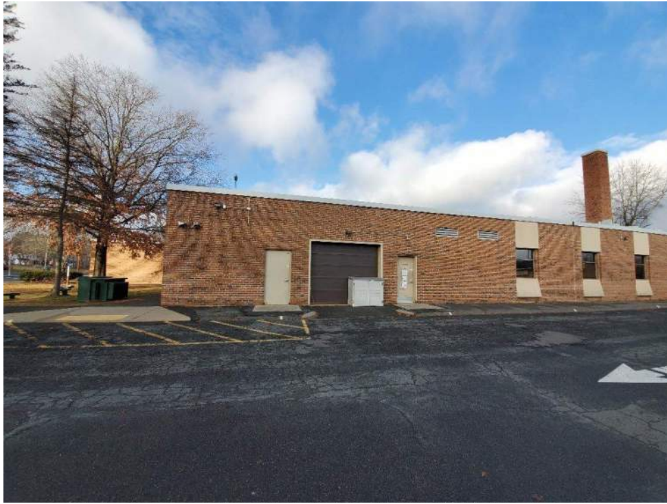
Photograph 13 – Fort River Elementary south side of building.
