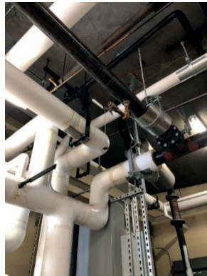
L & C - A set of 4" lines are extended to outside for temporary chiller hookup in case of chiller failure. R- boiler combustion air duct, which is no longer needed since the new boilers bring in outside air through individual ducts.
