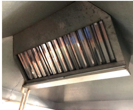
L & C- kitchen cooking line exhaust hood; the filters are Code- compliant panel type, but does not have Code mandated Ansul system. R- make up air is untreated (filtered or heated) through intake louver... understandably during summer it is hot and humid, but during winter the kitchen becomes freezing cold.
