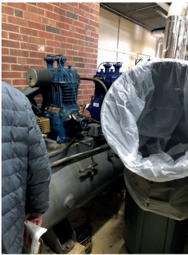
L - pneumatic control air compressor. C - pneumatic air dryer. R - Original pneumatic control panel.
