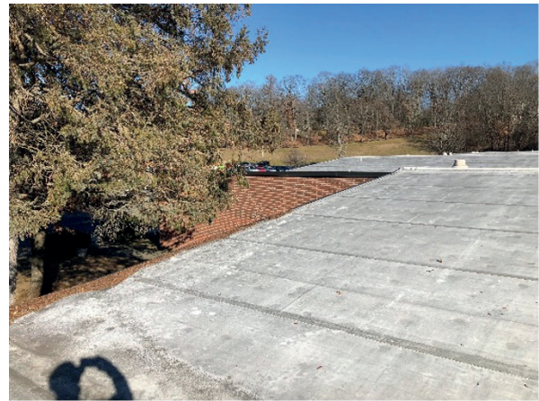
L- roof drain does not have overflow, are connected to internal conductor pipe, and to the under-slab piping to outside the building. R- roof edge does not have parapet.
