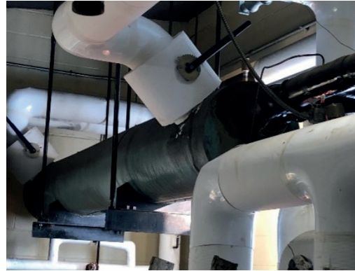
L - original 49 year old air cooled condensing unit on roof failed last year. C - note temporary electrical power cables on roof which were ran from the chiller to the rental chiller; nameplate was illegible, but thought to be 70-tons, which would be considered severely undersized by today's standard. R - chiller barrel (black above white pipes) inside right below.
