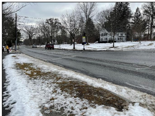
Photo 7: Approximately 200' separate the site exit driveway from the South East Street/Main Street intersection. Greater traffic volumes in the area could result in the queue from the signal extending beyond the driveway more frequently.
