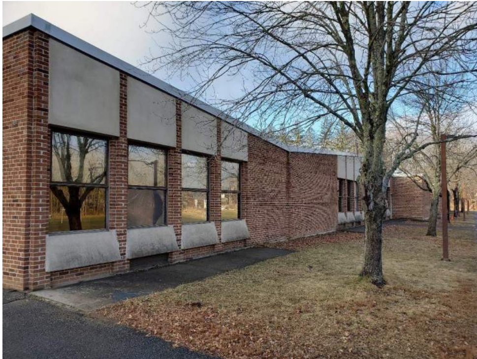
Photograph 5 – Fort River Elementary southeast side of building.
