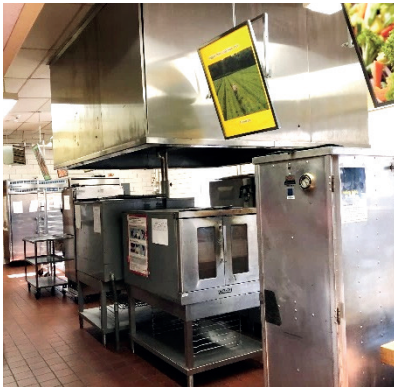
L & C- kitchen cooking line exhaust hood; the filters are Code- compliant panel type, but does not have Code mandated Ansul system. R- make up air is untreated (filtered or heated) through intake louver... understandably during summer it is hot and humid, but during winter the kitchen becomes freezing cold.
