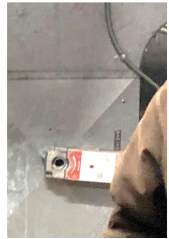
L - pneumatic control valve, here with ACM insulation sections removed. C - pneumatic control valve, here with remnants of encapsulated ACM insulation remaining. R - Electronic damper actuator.
