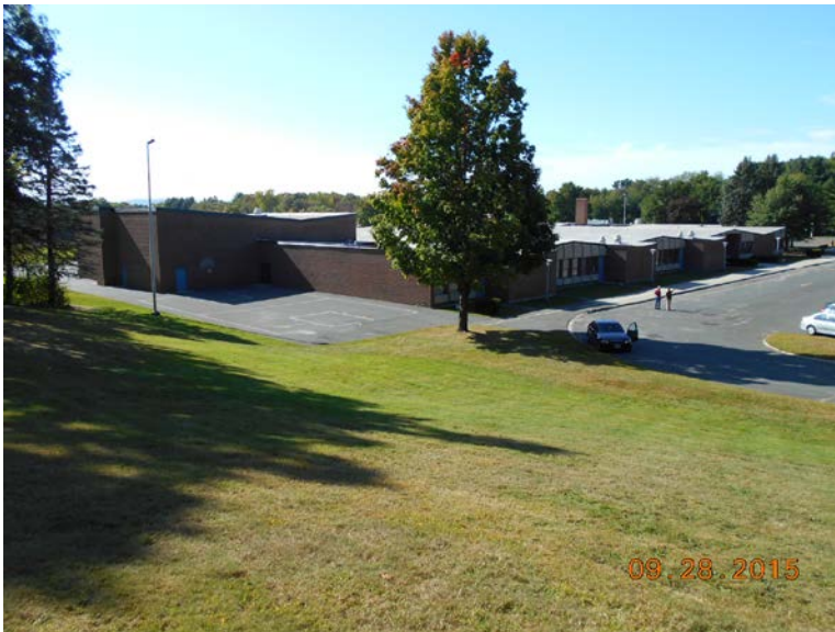
Photo #1: Site view from northeast
