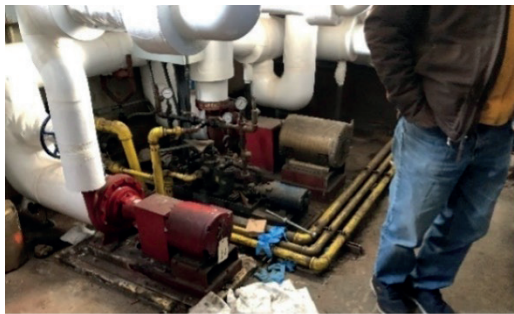
L - a 10,000-gallon underground fuel oil storage tank just outside the boiler room serves the space heating boilers; a 280-gallon underground tank serves the generator. C - Veeder-Root fuel oil level meter. R - fuel oil transfer pump set.
