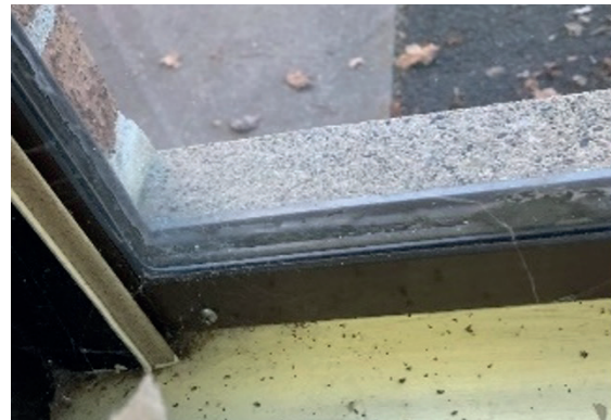
L - one of several courtyard / lightwell. R - original single pane glass were retrofitted with plastic panel inside, apparently not tight so the much debris is visible in the air space.
