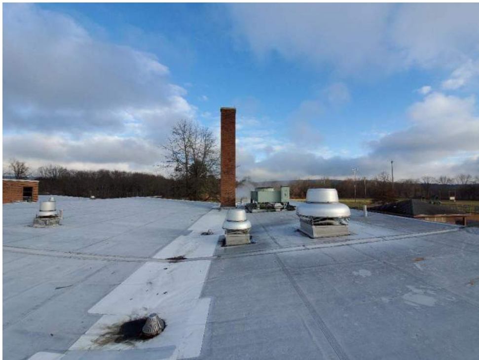
Photograph 14 – Fort River Elementary building roof.
