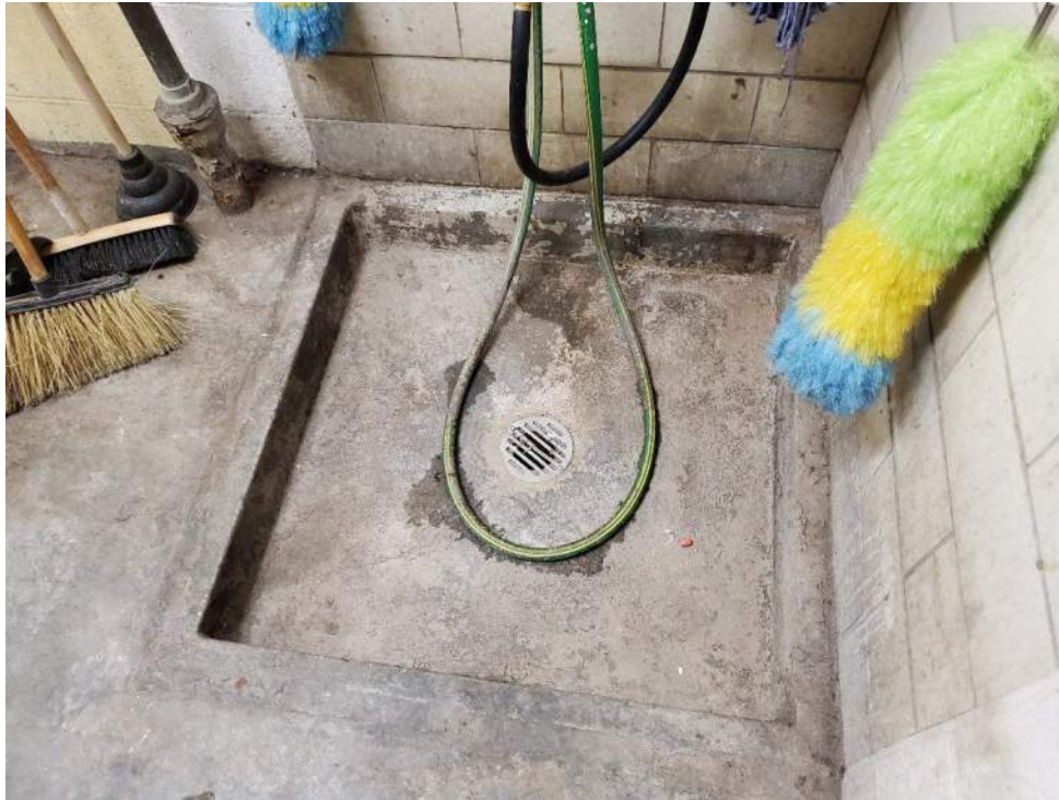
Photograph 17 – Custodial staff wash area with drainage.
